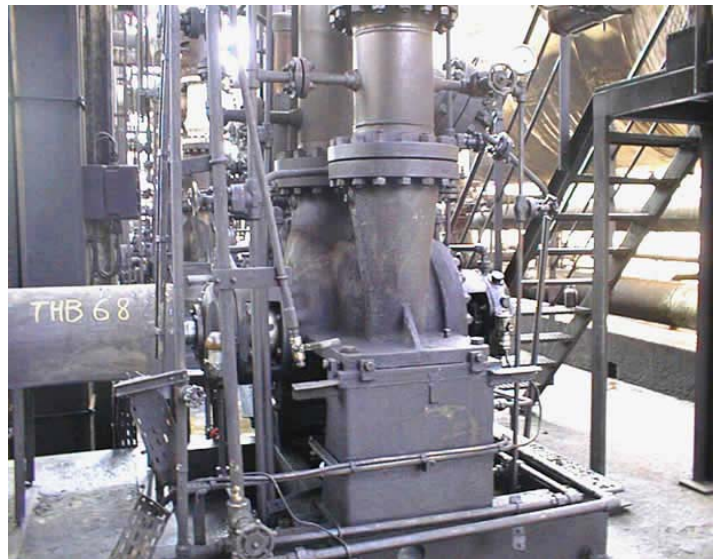
Figure 62: TT process pump, dual wheels between main bearings
