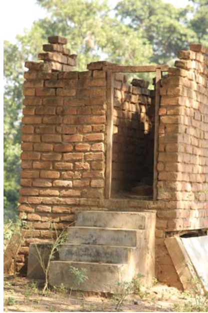
Figure 12.2 An abandoned latrine subsidized by Water For People in Chikhwawa.
