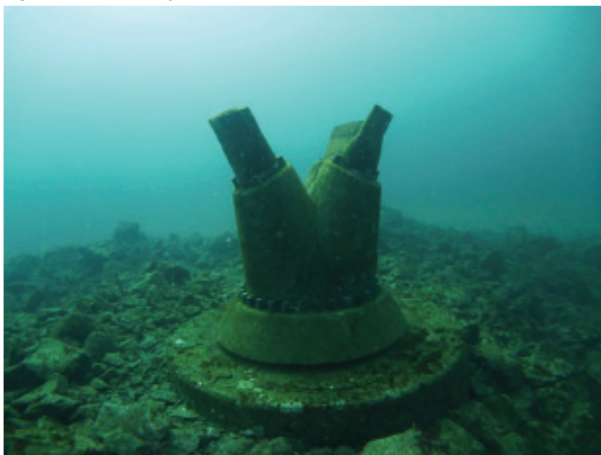
Figure 5. Discharge diffuser.
