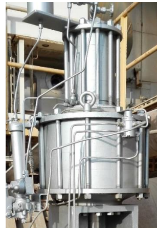
Figure 80: Double Cylinder Double Acting Actuator
