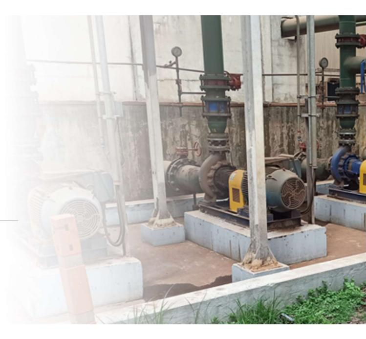
One of the biggest problems when designing a pump intake on a cooling tower sump is the risk of air intake in the pipeline or flow disturbances that **can damage or reduce the pump efficiency**.
