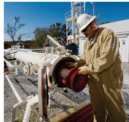
Fig 1. Loading a Cleaning Pig
