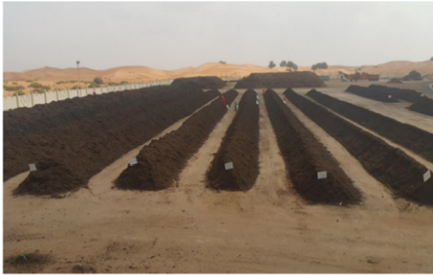
Figure 6-6: Example of Open-Air Windrow Composting at Al Ain Composting Facility
