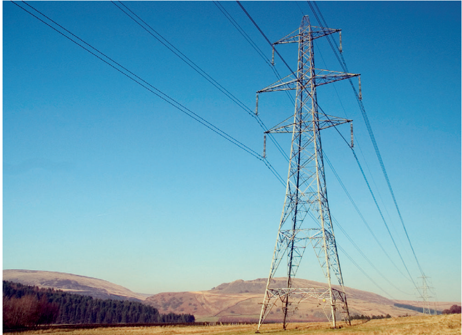
Figure 3.28 Transmission line steel pylon.
