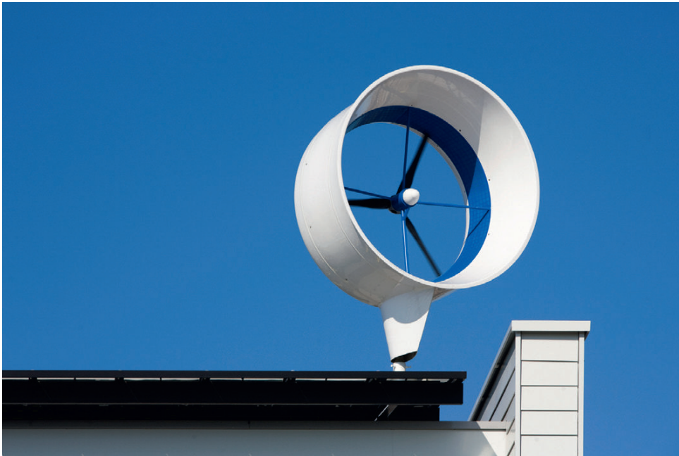
Figure 5.5 Small wind generator on a domestic property.
